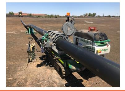
MCA owns and operates is own Polly Weld Machines with hire supply chain in place as required. Trained and ticketed operators
