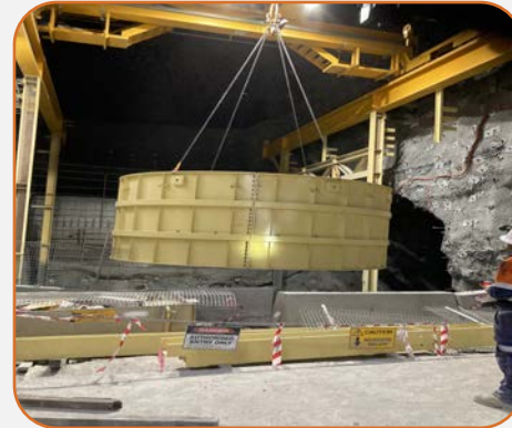
Lifted into position in shaft
