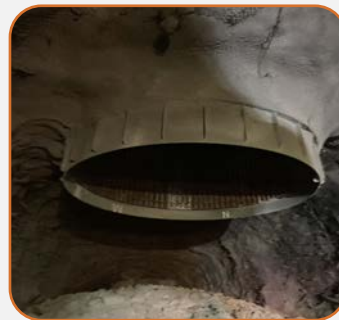
Created plug with 90 cubic meters of shotcrete
