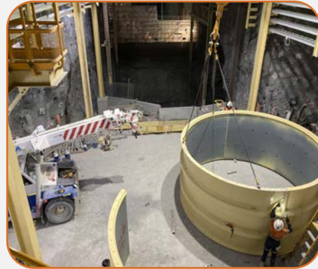
Assembled below ground
