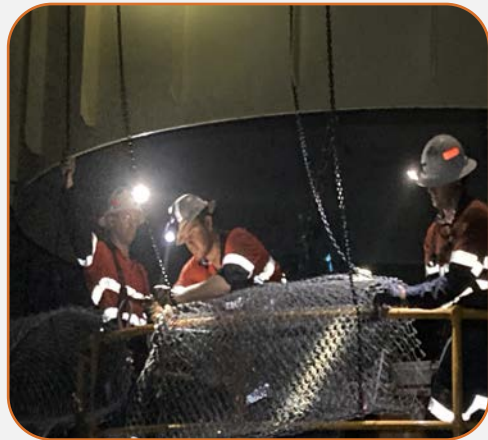
Installed scribing mesh
